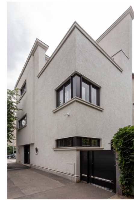
Realizarea elementelor arhitecturale și componențiale sacrificiate la execuția inițială / The newly built architectural and compositional elements, that were sacrificed when the house was initially built
