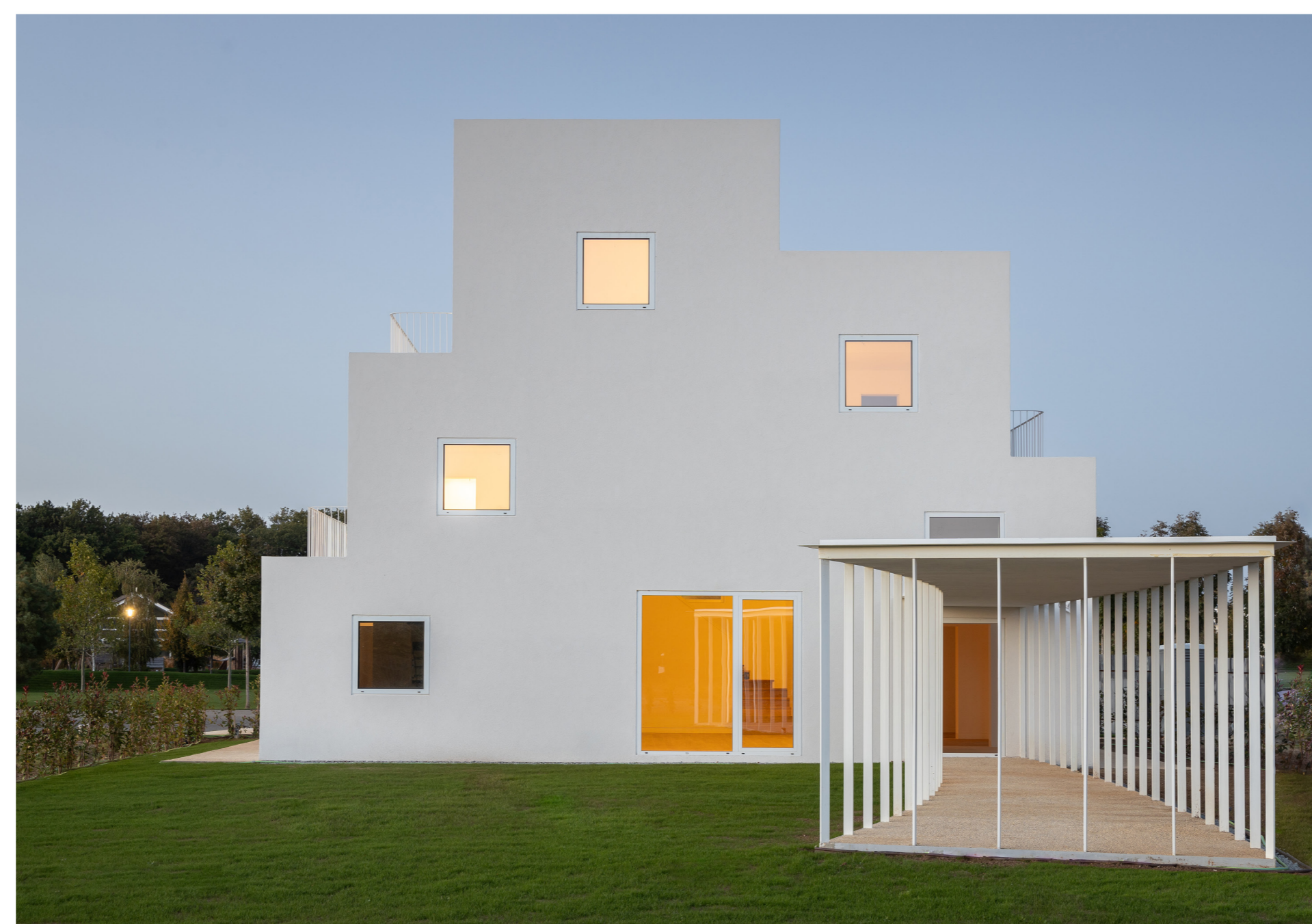
South façade (view from the garden)
