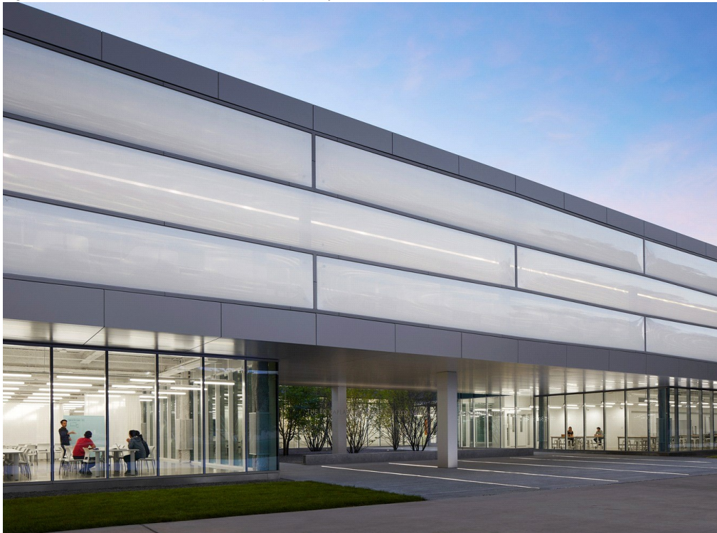
Figure4 – John Ronan Architects, Ed Kaplan Family Institute © Steve Hall
